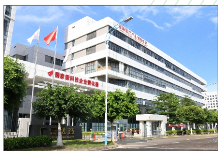
"WePure" Headquarter located in Guangdong
